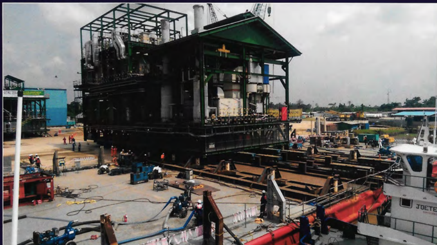
Skidding Operation in Progress
